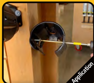
Use a 5" long bit to mount with screws
